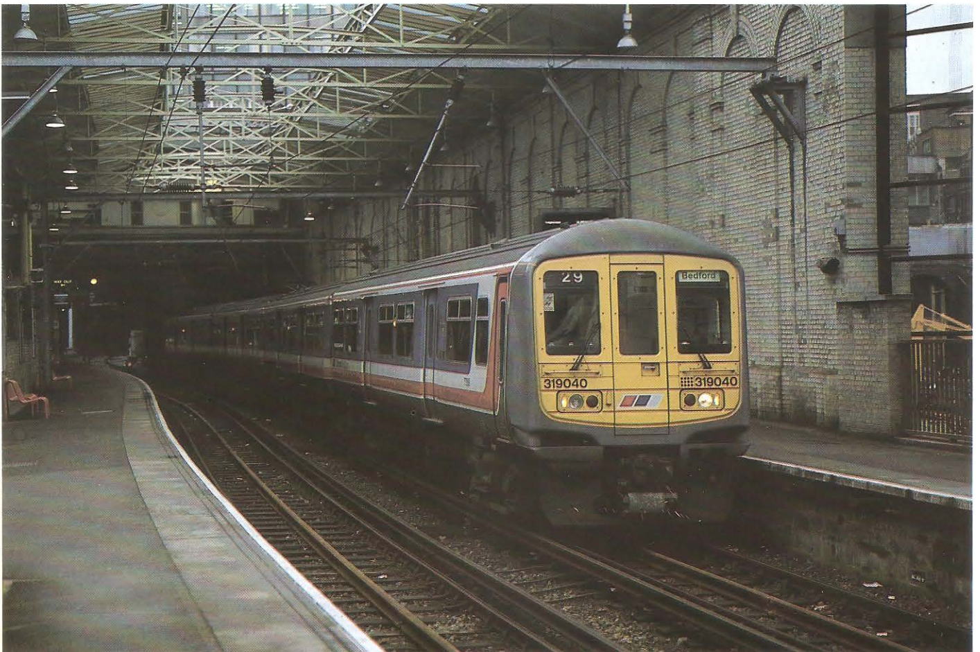
Change-over from 25kV ac to 750V dc (and vice versa) takes place at Farringdon station.
